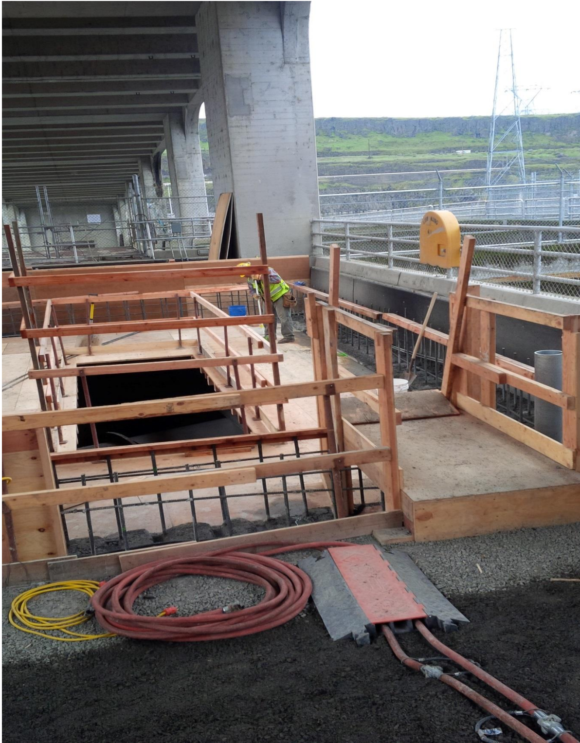
Finishing 7' valve room.
